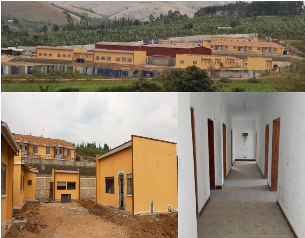
Figure 7: works progress at Ntungamo Beneficiation Centre is 90 % complete.
