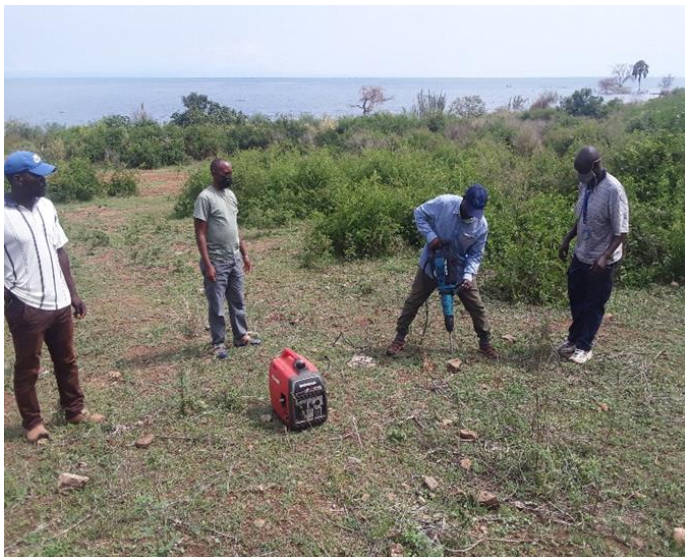
Figure 9: A portable hammer drill being tested
