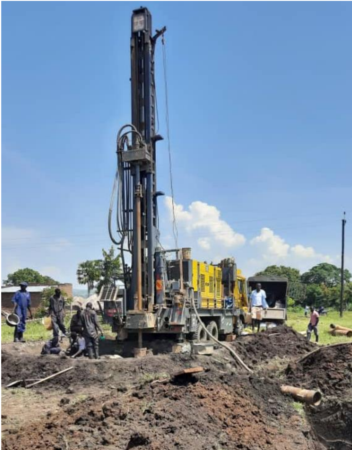
Figure 12: Drilling the first Temperature Gradient Holes at Panyimur.
