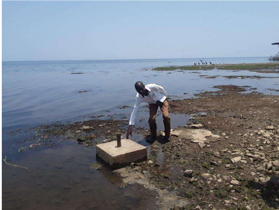
Figure 14: TGH (KB-2) reappearing on surface after the Lake waters retreated.
