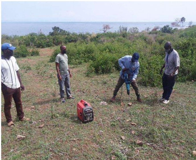
Figure 9: A portable hammer drill being tested
