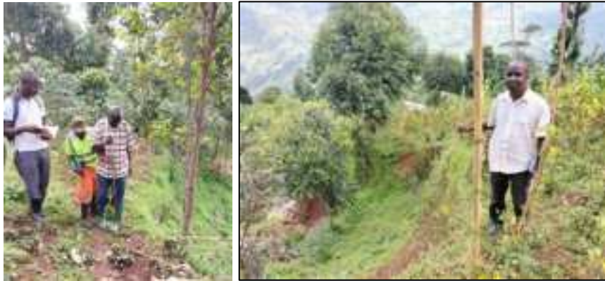
Figure 23: The team assessing the extent of cracks at Elgon Sub County
