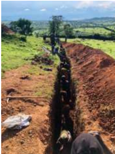
Figure 8 Trench 3 excavation in Lwensakala
