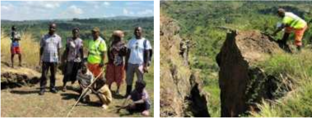
Figure 21: GSD field team on Kerate rack (L). The boy on the right (with RED Short) is standing on a hanging rock. Note the relative with of the widening crack.
